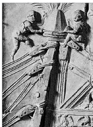
Fig. 6 Details of the dangling ropes and metallic pulley blocks. (© Musei Vaticani)
